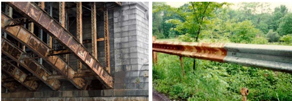
Figure 7. Example of bridge and highway structures getting corrosion ( www.galvanizeit.org ).
