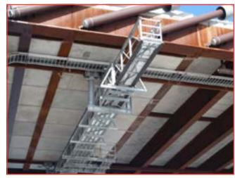
The Mississippi River Bridge Traveler is the newest innovation in high structure inspection and repair. Whether used on a bridge, pipe support rack, or utility structure, the "Traveler" provides a safe and efficient platform for inspection and repair. Suspended under a Mississippi River Interstate Bridge and hundreds of feet above the River, corrosion is a monumental safety concern. Hot-dip galvanizing provides peace of mind for inspectors and repairmen.
