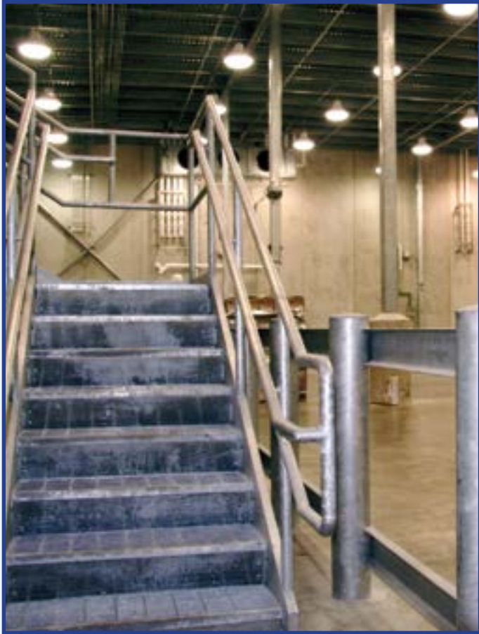
The Quick Chill Cooler expansion was hot-dip galvanized to help meet USDA food processing requirements and to withstand the extreme cold environment.
