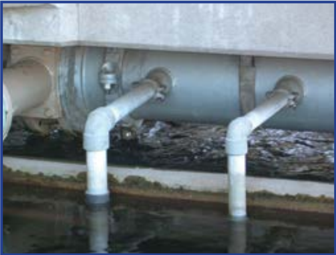
This water treatment facility was galvanized to protect steel from the many corrosive properties of ground water.
