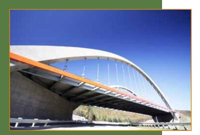
he suspended Stoneham Arch Bridge is an aesthetically pleasing solution to a unique site requirement. The choice of hot-dip galvanizing was preferred by the engineer because of its durability and cost compared to Cor-Ten steel in this highly corrosive environment. The resulting bridge is a beautiful and cost-effective marriage between structural steel and reinforced concrete.
