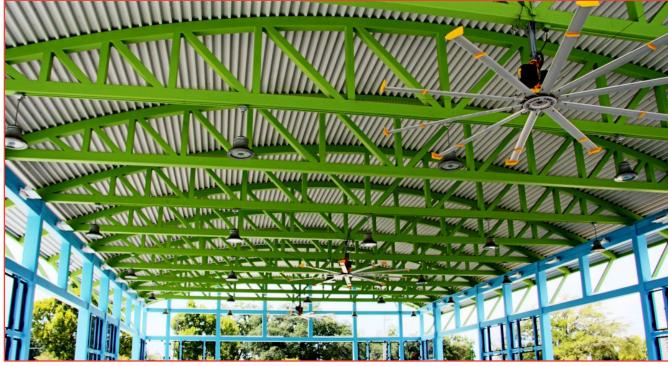
The engineer, fabricator and galvanizer worked together to provide venting and drainage to the tubular components especially since some required progressive dipping. The galvanizer took extreme care to avoid distortion and provide the smooth surface needed for painting.
