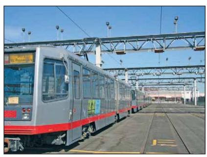
money on constant repairs and touch-up. As the centenary trusses, angles, and beams are critical to keeping the electrical cables and lighting supported, galvanizing will provide uninterrupted service for the maintenance facility.
