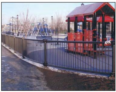
The Massachusetts Port Authority wanted to protect the steel in Logan Park and knew it needed a strong coating because of the park's proximity to the water and the aggressive Massachusetts winter. The Port Authority decided on a duplex system of hot-dip galvanizing and paint because of its superior corrosion protection.
