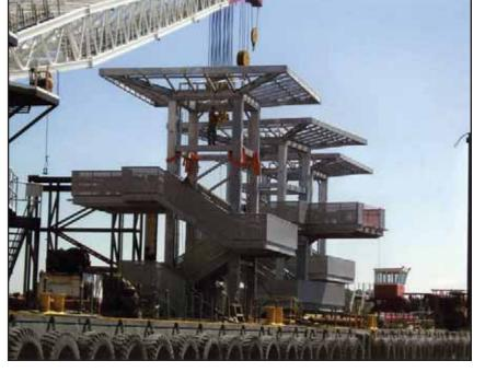
demanding project schedule – and galvanizing accommodated this requirement. The towers were assembled in an offsite location and subsequently transported to the site after being fully erected. A large 500 foot water crane lifted the towers onto the imposing iron maiden. Galvanized steel will keep the Intrepid structurally sound and ship-shape for generations to come.
