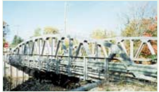
Webb Avenue Bridge
