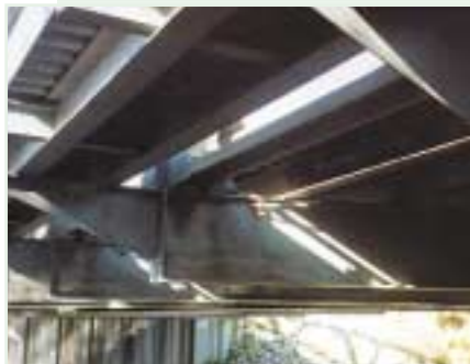
View of the underside of the bridge
