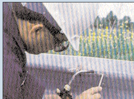
Zinc solders provide the best color and aesthetic match between the repaired area and the original galvanized surface.
