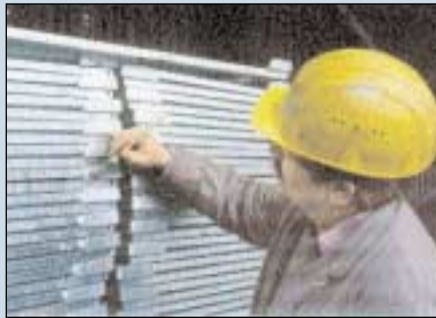
Zinc rich paints provide the simplest method of repair to damaged galvanized coatings. They are easy to apply, as shown above.
