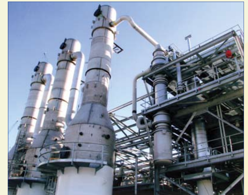
Many Ethanol plants originally painted for corrosion protection are now being retro-fitted with hot-dip galvanized steel after just a few years. As new ethanol plant production has slowed, this area continues to grow.
