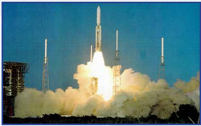
The lightning mitigation system towers were galvanized to withstand the extreme high temperatures at launch.
