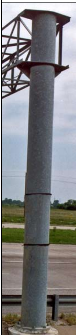
Galvanized sign structure
