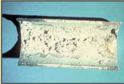
FIGURE 22: FLUX INCLUSIONS FROM INTERIOR OF PIPE (REJECTABLE)
