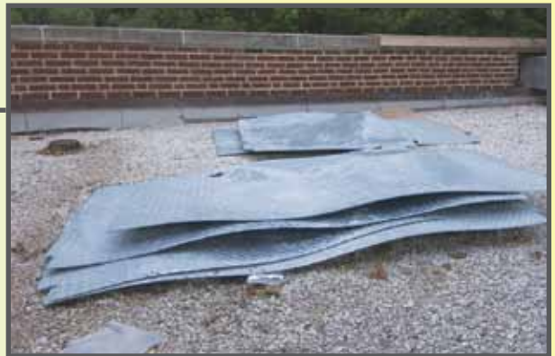
FIGURE 17: DISTORTION (ACCEPTABLE)
