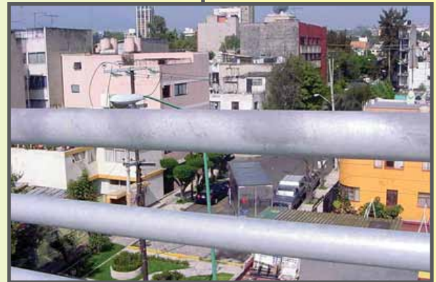
FIGURE 11: GRAY COATING DUE TO PROCESSING (ACCEPTABLE)
