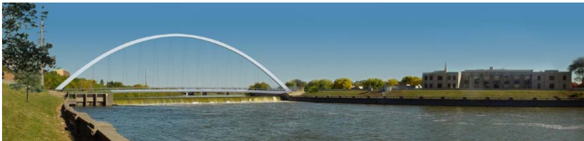
Center Street Pedestrian Bridge, Courtesy of Stanley Consultants, Inc., Des Moines, Iowa.
