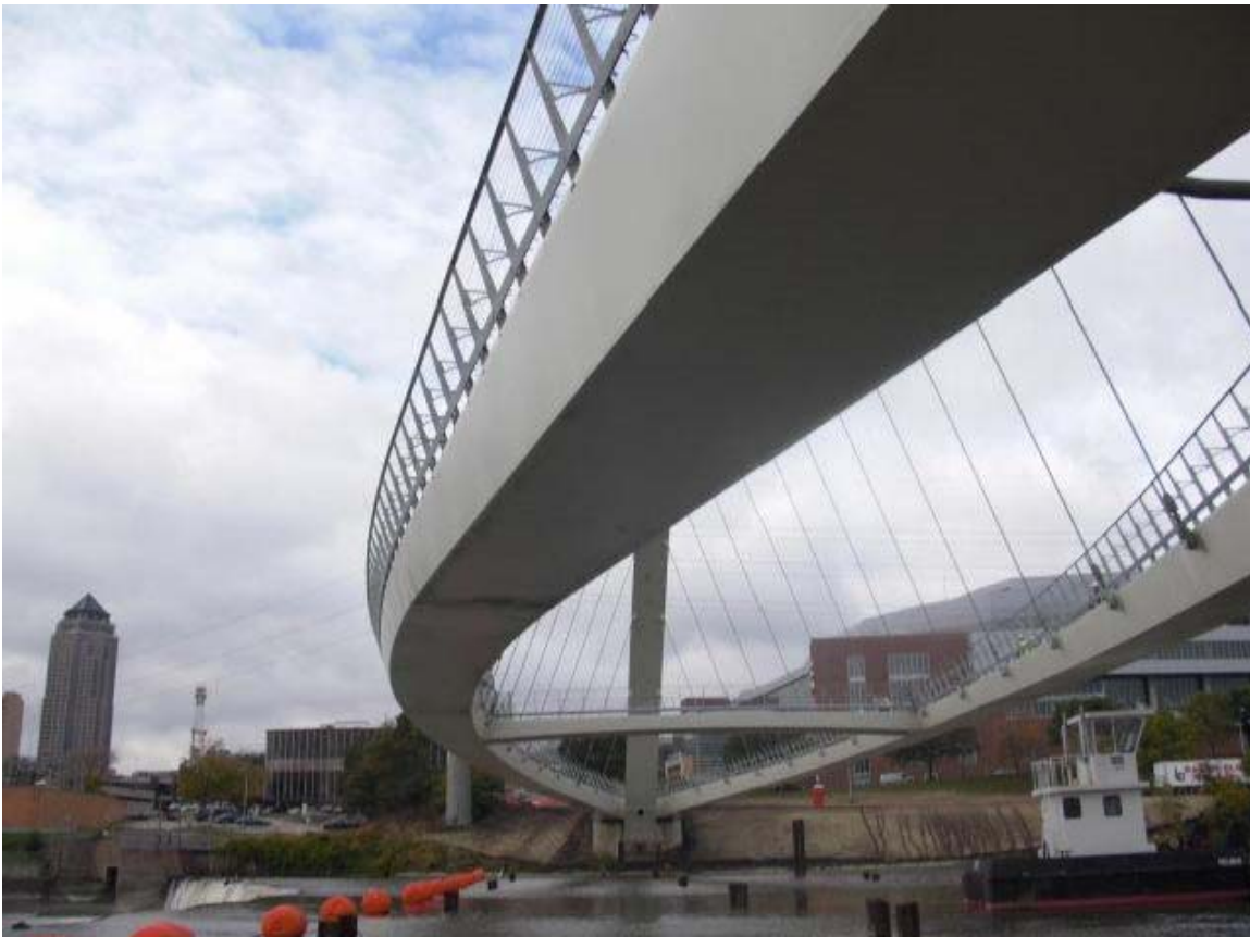
Center Street Pedestrian Bridge, Courtesy of Stanley Consultants, Inc., Des Moines, Iowa.
