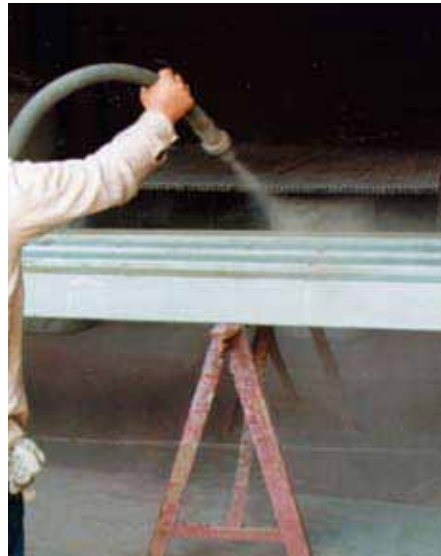
Sand blasting pre-treatment
